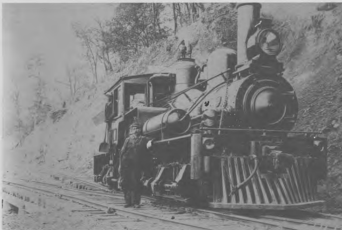
This locomotive named "Old Jeb" was used in the building of the Cheat Lake Dam, 1912-1913.
