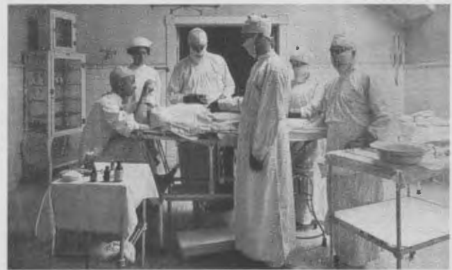
Operating Room of the McKendree Miners' Hospital, circa 1914.
